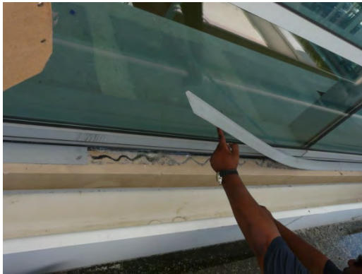
Photo #1920264. Sill trim panel visibly misaligned and showing excessive deflection when touched by hand.
