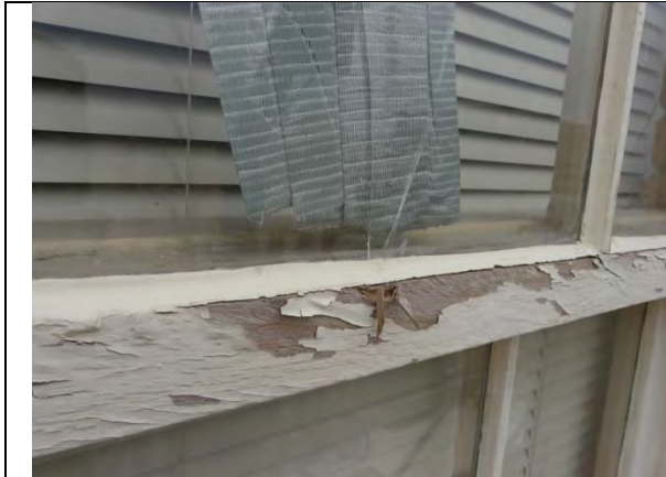
1. An unusual impact signature at the meeting rail, with forces transferred via its glazing compound to the glass pane, resulting in its stress breakage. The peeling coating is a preexisting condition. Window #60, 12/17/2014
